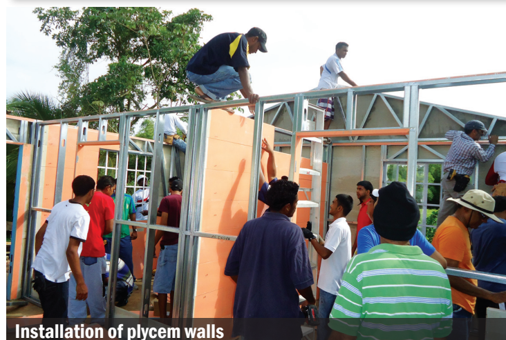
Volunteers set up the steel frame, Trinidad
